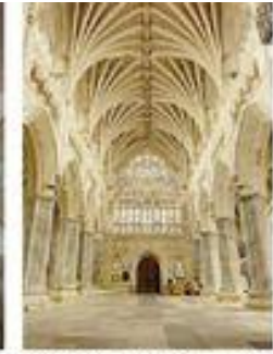
rib vaulting, Exeter Cathedral Exeter, UK (architect unknown, 1400)
