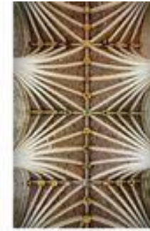
rib vaulting, Exeter Cathedral Exeter, UK (architect unknown, 1400)
